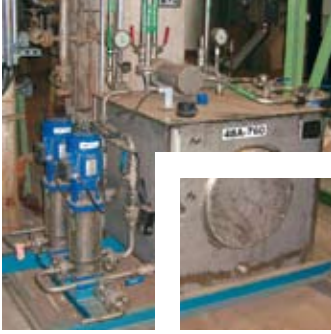
SPA 4002 for supplying 12 agitator seals on thin-film evaporators at DOMO Caproleuna.
