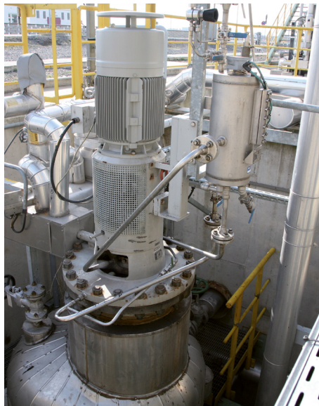
Agitator seal with TS-system
