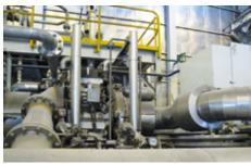
A type **DGS30** gas-lubricated mechanical seal is used to seal a compressor in BASF's synthesis gas plant in Shanghai, China. Nitrogen-buffered **Espey WD400** floating ring seals seal the bearings. The process medium is carbon dioxide. Operating conditions:  $p_1$  (dynam.) = 18.5 bar (268 PSI); t = 70 °C (158 °F); n = 25,750 min<sup>-1</sup>.
