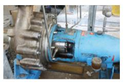
Centrifugal pumps at Polymer-Latex GmbH in Marl, Germany, are successfully sealed with **Cartex-DN** type seals. The process medium – a latex dispersion – represents a challenge for the seal. The **FLC200** flow rate control unit supplies and flushes the seal.
