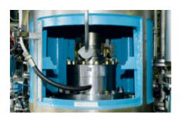
Wacker Chemie AG in Burghausen, Germany, seals a number of top-drive high pressure reactors for polymer dispersion manufacturing with **HSHLV-D** type high pressure seals with cooling flange. A shared buffer system supplies all the seals. Operating conditions:  $p_1 = \text{vacuum} \dots 100 \text{ bar} (1,450 \text{ PSI}); t = \dots 100 \text{ °C } (212 \text{ °F}); n = 25 \dots 100 \text{ min}^{-1}.$
