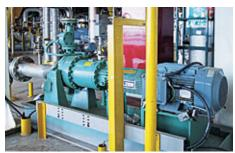
Sealing of a centrifugal pump for the manufacture of aromatic compounds at Shell in the Netherlands. The high drive power of 75 kW makes it necessary to apply a high efficiency **NMB-22P-9R-35-ND** magnet coupling. This uniquely efficient magnetic coupling drastically reduces power losses and the associated heat generation. Operating conditions:  $p=35 \text{ bar } (508 \text{ PSI}); t=20 \text{ °C } (68 \text{ °F}); \\ n=990 \text{ min}^{-1}.$
