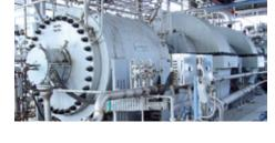
Sealing a coolant compressor at the Yeochun NCC Company in Korea with a **PDGS10** – a gas-lubricated multiple mechanical seal in tandem arrangement. The medium to be sealed is ethylene. Heat tracing at temperatures down to –100 °C (–148 °F) is unnecessary due to the application of a special dynamic secondary sealing element.
