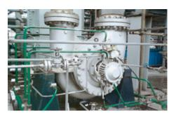
Fujian Refining & Petrochemical Co., Ltd. in China applies a BB2 pump for propane de-asphalting. The shaft seal is an EagleBurgmann **SHV1/102-PTA1/2**. Configuration 2CW-CW, piping plans 21+52. Operating conditions: p=73 barg (1,059 PSIG); t=165 °C (329 °F); n=2,970 min<sup>-1</sup>.
