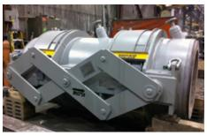
EagleBurgmann **high-end standpipe expansion joint** installed in a refinery in Texas, USA. Operating conditions:  $p = \dots 6.89$  bar (100 PSI); t = 510 °C (950 °F); t = 1,170 mm (46"). Medium: flue gas.
