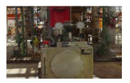
**H75KF-D1/130** back-to-back dual seals with supply system **SP09030/M012-D1** to API 682 Plan 53 have been successfully sealing the shafts of Pacific between bearing pumps since 2004. The system is located in the CRP refinery of Petroleos De Venezuela S.A. Operating conditions: p=4 barg (58 PSIG); t=200 °C (392 °F); n=3,600 min<sup>-1</sup>; d1=104.1 mm (4"). Media: naphtha, gasoil +3% H<sub>a</sub>S.
