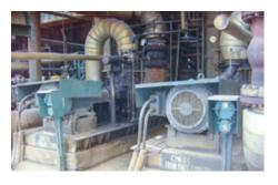
EagleBurgmann seal type **Y14D64TC** with supply system to API 682 Plan 11 and 62 running successfully in a KEPL centrifugal pump in the distillation unit of Kochi Refineries Ltd., India, since 2002. Operating conditions:
