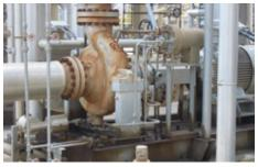
**MFLWT80F2/85** mechanical seals with a **WEL** air fin cooler to API 682 Plan 21, installed in a bottom pump-around pump from Sulzer in the distillation unit of the Sohar refinery in Oman. Operating conditions: p=...4.19 barg (60 PSIG); t=278 °C (532 °F); n=1,475 min<sup>-1</sup>; d1=68 mm (2.68"). Medium: gas oil.
