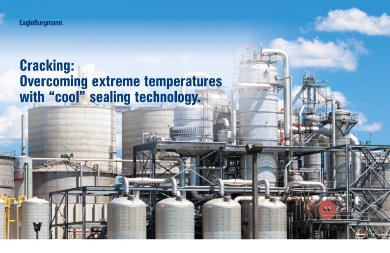
The fraction of crude oil which cannot be distilled further is then cracked. In this process, long chain molecules are split into smaller molecules under pressure and temperature in order to generate additional short-chain hydrocarbons such as gasoline, diesel or kerosene.
