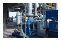
Stripper reflux pumps within the naptha hydro treater unit of the ENOC refinery in Dubai are fitted with EagleBurgmann **H75VKS20/105** mechanical seals and supplied to API 682 Plan 11. Operating conditions:  $p=11.77 \text{ bar } (25 \text{ PSI}); t=43 \text{ °C } (109 \text{ °F}); \\ n=1,485 \text{ min}^1; d1=80 \text{ mm } (3.15").$  Media: hydrocarbons.
