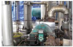
Boiler feed water pumps in the hydrogen unit of the Turkish Tüpras Kirikkale refinery are equipped with EagleBurgmann **SHPV2/64** seals and supply systems to API 682 Plan 02 + 23. Operating conditions: p = 43 bar (624 PSI); t = ... 282 °C (540 °F); n = 1,470 min<sup>-1</sup>; d = 58 mm (2.28"). Medium: boiler feed water
