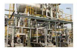
The ENI refinery in Sannazzaro De' Burgondi, Italy, operates a Finder centrifugal pump in its gasification unit. The pump is sealed by EagleBurgmann **HRKS4-DF/58** mechanical seals. Operating conditions:  $p=16.08\ldots19.93$  bar (233 ... 289 PSI); t=238 °C ... 263 °C (460 °F ... 505 °F); n=2,955 min<sup>-1</sup>; d=80 mm (3.15"). Medium: carbon slurry.
