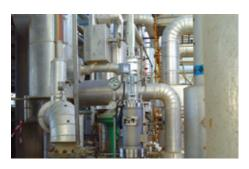
EagleBurgmann mechanical seals are installed in demethaniser reboiler pumps from Thompson Byron Jackson at the Santos-owned Moomba gas plant in South Australia. EagleBurgmann solved the challenges with its seal type **H75KF-D** and a supply system to API 682 Plan 53C. Operating conditions: p=36 bar (522 PSI); t=-20 °C ... +38 °C (-4 °F ... +100 °F); n=1,480 min $^{-1}$ . Media: light hydrocarbons.
