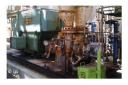
In the alkylation plant of the refinery of Salina Cruz, Oaxaca, Mexico, our **H74-D/85** functions as a dual seal for between bearings pumps from Byron Jackson. Operating conditions: p=9.61 bar (139 PSI); t=42.3 °C (108 °F); n=3,550 min<sup>-1</sup>; d1=79.38 mm (3.12"). Media: hydrocarbons + hydrogen fluoride.
