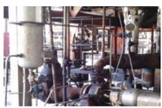
In the distillation unit of a Mexican refinery in Salina Cruz, Oaxaca, EagleBurgmann metal bellows seals type **MFLWT80/75** seal the shafts of Sulzer horizontal pumps. Operating conditions: p = ... 9.42 bar (137 PSI); t = 175 °C (347 °F); t = 3.560 min<sup>-1</sup>. Media: hydrocarbons
