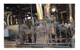
Kochi Refineries Ltd., India applying in their visbreaker unit EagleBurgmann metal bellows seals **Y14D52C** with a supply system to API 682 Plan 32 + 62 in an Ebara centrifugal pump. Operating conditions: p = ... 8.9 bar (129 PSI); t = 247 °C (477 °F); n = 1,780 min<sup>-1</sup>; p1 = 75 mm (2.95"). Medium: vacuum residue.
