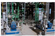
In the ENOC refinery in Dubai, U.A.E., LPG pumps are sealed by EagleBurgmann **H75VKS20/85** dual tandem face-to-face mechanical seals. Applied API piping plans: 11 + 53B. Operating conditions: p = 17.75 bar (257 PSI); t = 43 °C (109 °F);  $t = 2,950 \text{ min}^{-1}$ ; t = 60 mm (2.36"). Media: hydrocarbons.
