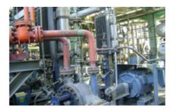
For a KSB pump installed in the delayed coker unit, the Indian Panipat refinery applied EagleBurgmann pusher seals **LL9DTUU** in tandem arrangement. Operating conditions: p=23.5 bar (340 PSI); t=40 °C (104 °F); n=2,900 min<sup>-1</sup>; d1=58 mm (2.28"). Media: hydrocarbons.
