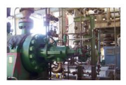
**H75KF-D1/130** back-to-back dual seals with supply system **SP09030/M012-D1** to API 682 Plan 53 have been successfully sealing the shafts of Pacific between bearing pumps since 2004. The system is located in the CRP refinery of Petroleos De Venezuela S.A. Operating conditions: p = 4 barg (58 PSIG); t = 200 °C (392 °F); n = 3,600 min<sup>-1</sup>; d1 = 104.1 mm (4"). Media: naphtha, gasoil + 3 % H<sub>a</sub>S.
