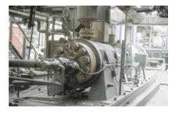
EagleBurgmann **MFLWT80S3/90** sealing Byron Jackson pumps supplied to API 682 Plan 02 + 54 by an EagleBurgmann **SPA 3020/A22** supply system. Operating conditions:  $t = 332 \,^{\circ}\text{C}$  (630  $^{\circ}\text{F}$ ); p = 8.5 bar (123 PSI). Medium: residual oil.
