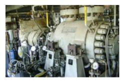
A high pressure dry gas seal EagleBurgmann type **PDGS2.1/130** seals a Bhel compressor in the hydrocracker unit of the Panipat refinery in India. Operating conditions: p = ... 179 bar (2596 PSI); t = 160 °C (320 °F); d1 = 112 mm (4.41"). Media: H2 + CH4, N2.
