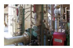
Since 2001, PDVSA (Petroleos de Venezuela) has been using EagleBurgmann seals type **H75K/110** with supply system **TS6050** to API 682 Plan 52 in a Sulzer between bearings pump. Operating conditions: p = ... 4 bar (58 PSI); t = 52 °C (126 °F); n = 3,560 min<sup>-1</sup>; d1 = 80 mm (3.15"). Media: aromatic hydrocarbons.
