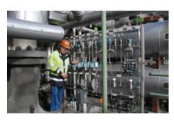
For a MAN Turbo compressor at Shell Godorf, Germany, EagleBurgmann has supplied a **DGS20/113** dry gas seal together with a **SMS** seal management system. The compressor is operated in the gas processing section of the plant. Operating conditions: p=...30 bar (435 PSI); t=-20 °C ... 180 °C (-4 °F ... 356 °F); t=-9.811 min<sup>-1</sup>; t=-9.811 m
