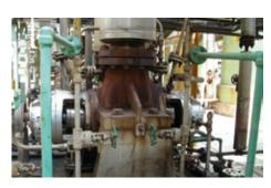
EagleBurgmann **LL9DTUU** dual mechanical seals are applied to seal a Sulzer pump of a catalytic cracking unit operated by Chennai Petroleum Corporation Ltd. in India. Operating conditions: p = ... 13.73 bar (199 PSI); t = 40 °C (104 °F); n = 2,965 min<sup>-1</sup>; d1 = 70 mm (2.7"). Media: hydrocarbons.
