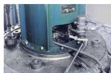
EagleBurgmann HGH210/225-E1 are installed in the main cooling water pump at the KNG power plant in Rostock. Operating conditions: p = 2.25 bar (23.63 PSI);  $t = 25 \degree C (77 \degree F)$ ;  $n = 490 \text{ min}^{-1}$ ; medium: brackish water with sand.
