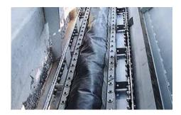
**Fluastal** expansion joints (9 x 5 m) made of special fabric are installed in a flue gas duct at the EGAT Wang Noi power plant in Thailand. Operating conditions: p = 0.074 bar (1.07 PSI); t = 580 °C (1,076 °F).
