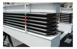
**Expansion joints** with specially shaped edges are installed in an air preheater at East Kentucky Power in the US. Operating conditions:  $p = 0.07 \dots 0.24$  bar (1.02 ... 3.48 PSI);  $t = 34 \dots 540$  °C (640 °F ... 1,004 °F).
