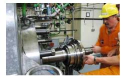
An EagleBurgmann **SHV1/165-E2-Q** mechanical seal is applied as shaft seal on the main feedwater pump at the E.ON Isar I nuclear power plant in Germany. Operating conditions: p = 20 bar (290 PSI); t = 185 °C (365 °F); n = 5,730 min<sup>-1</sup>.
